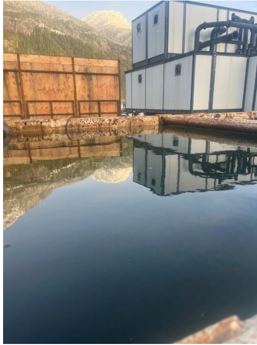
No visible sheen on discharging water
