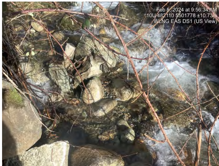
Photo: 1 Location: Downstream Description: DS location - US View
