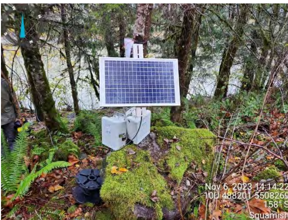
Photo 3. Location: Squamish River SQU US1 View: Northwest Caption: Solar panel setup moved to area with less vegetation for more direct sunlight.
