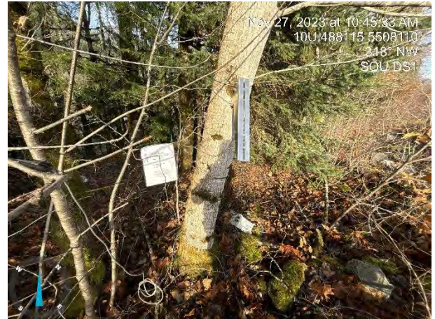
Photo 4. Location: Squamish River SQU DS1 View: Northwest Caption: Solar panel and one telemetry unit stolen. Remaining telemetry unit on ground.
