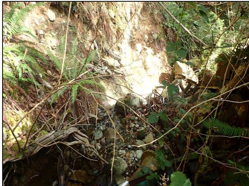
Photo 4 View downstream at bend approximately 30 m upstream of the proposed discharge location, showing instability and erosion on north slope. (October 4, 2019).
